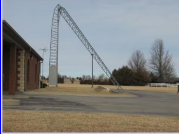
Wind-damaged tower in Princeton, Kansas Photo by Sherry Durst
