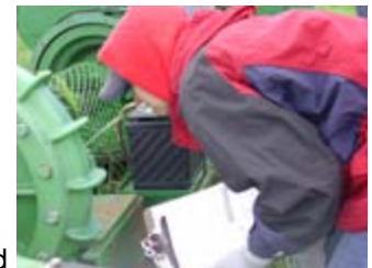
Ebert takes a closer look at an irrigation pump.
